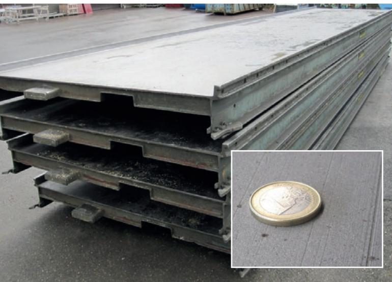
*Poor quality of a pallet formwork surface before renovation: deep scoring and uneven formwork surface; poor paintwork*
